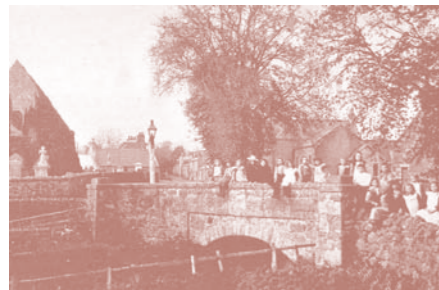
The old Neil bridge.
